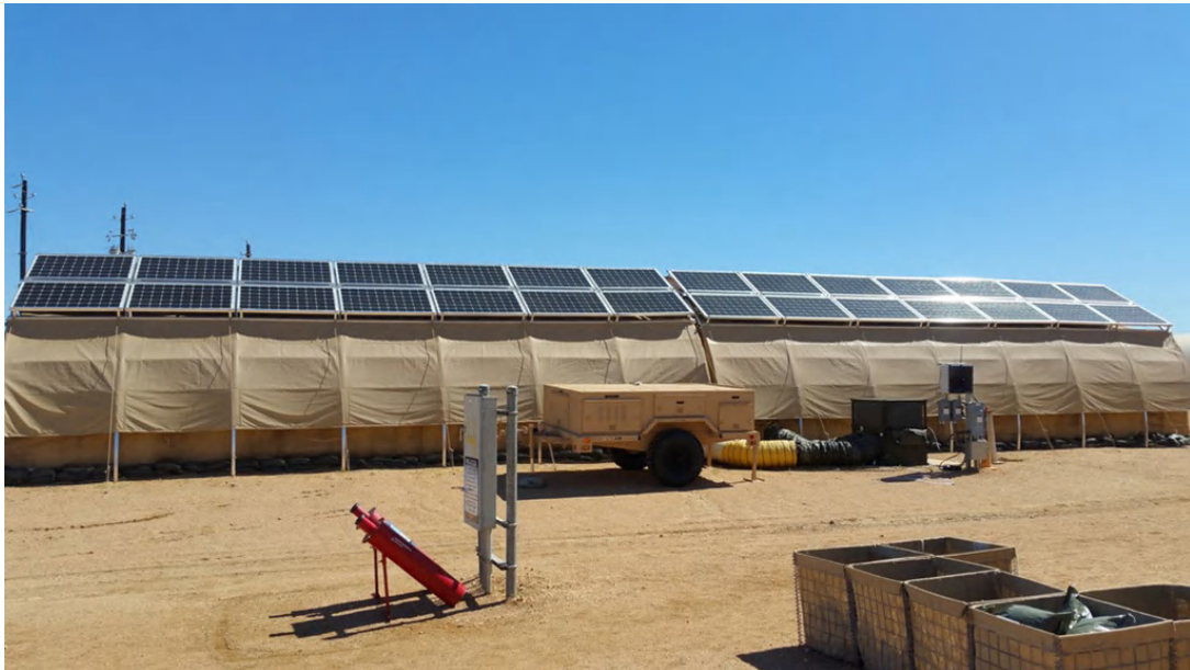
Figure 12 Monocrystalline silicon solar panels are placed for energy production at Lackland AFB, Texas
