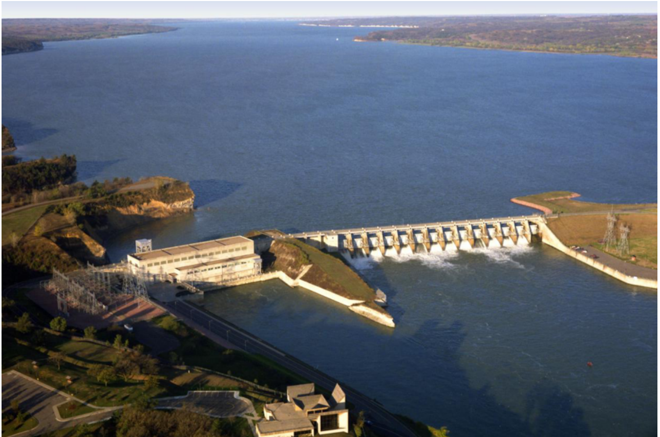
Figure 4. Gavins Point Dam and its 14 spillway bays, retrieved from U.S. Army Corps of Engineers
