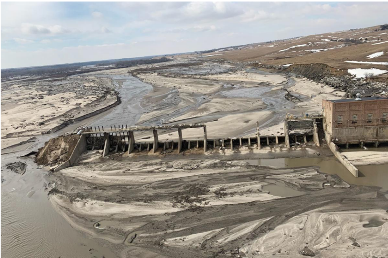
Figure 3. Spencer Dam after its failure, retrieved from Nebraska State Peter Rickett Governor Office
